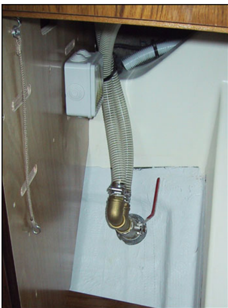
Thru-hull fitting with valve, draining of the sink
