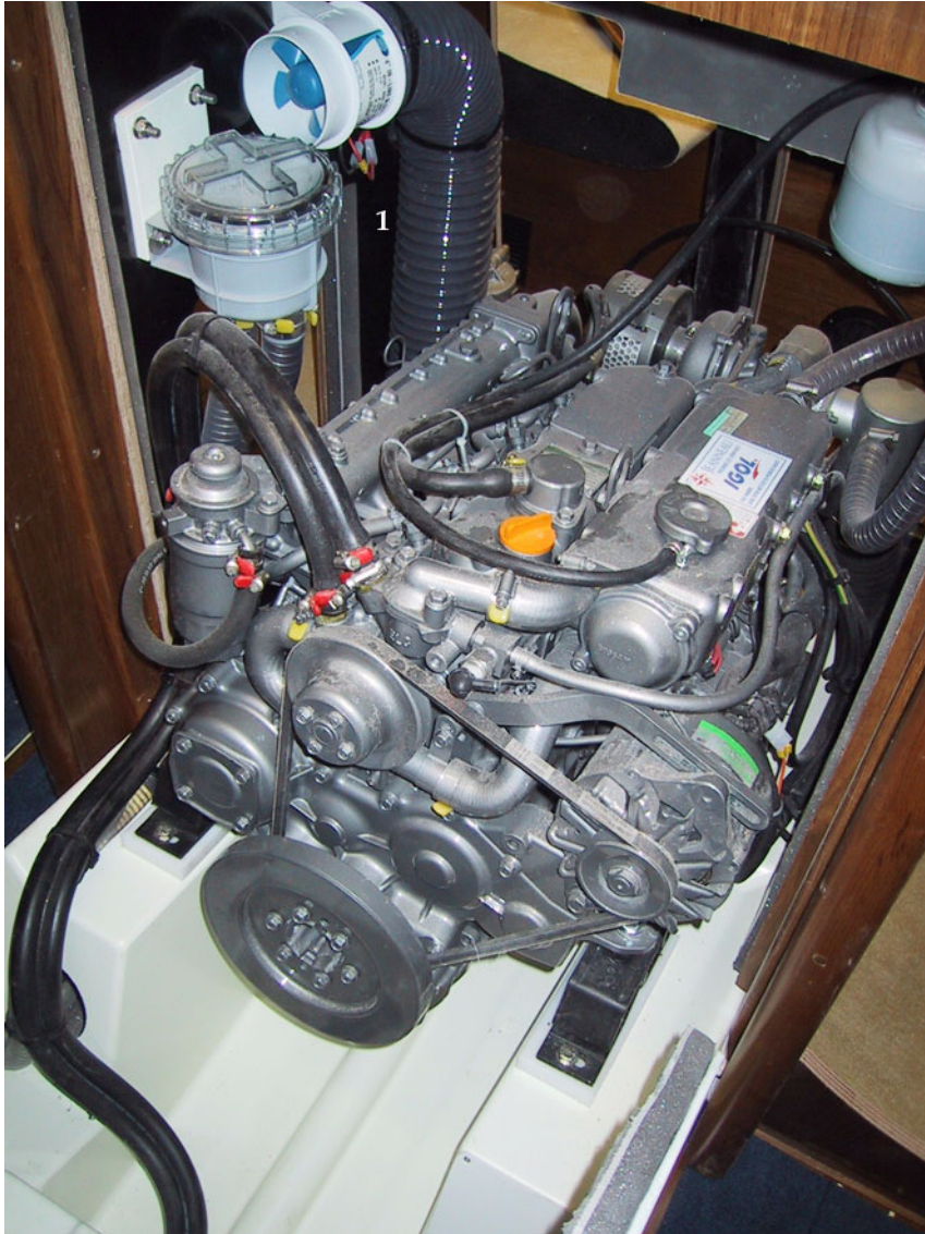
1. Filter for engine cooling water
