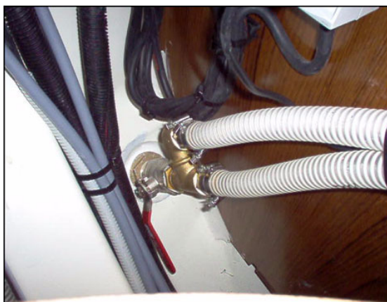
Thru-hull fitting with valve, draining of the sink
