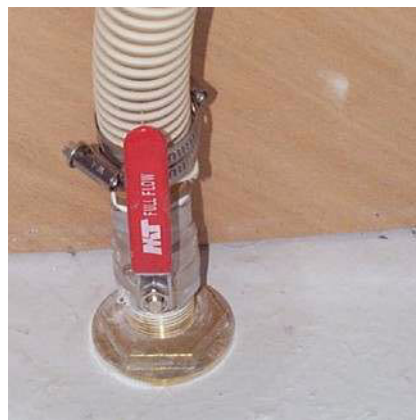
Thru-hull fitting open
